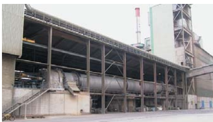
Holcim Siggenthal, Switzerland
